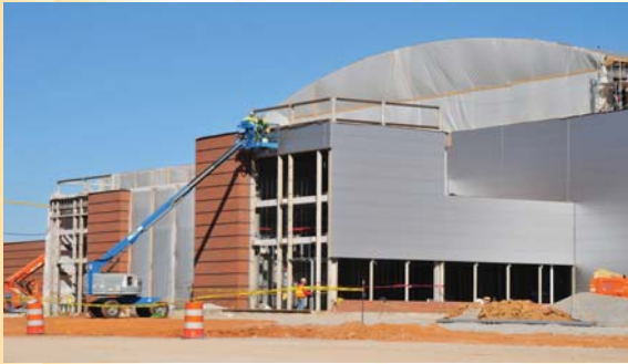
Solar Center construction is ongoing and anticipated office occupation is spring 2011.
